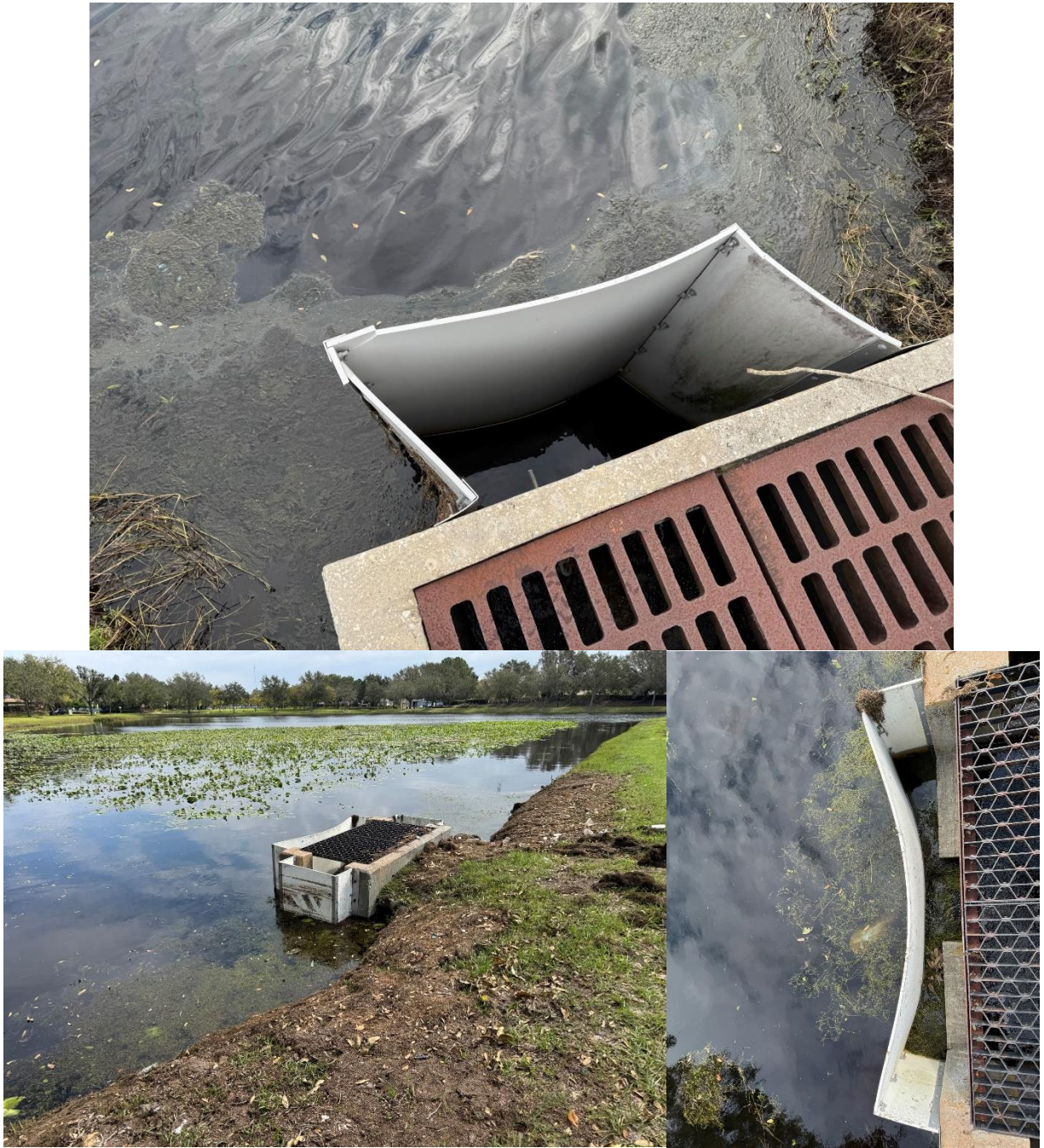
Photo 2 – Displays images from Pond 011 and Pond 14 with the bent skimmers.
