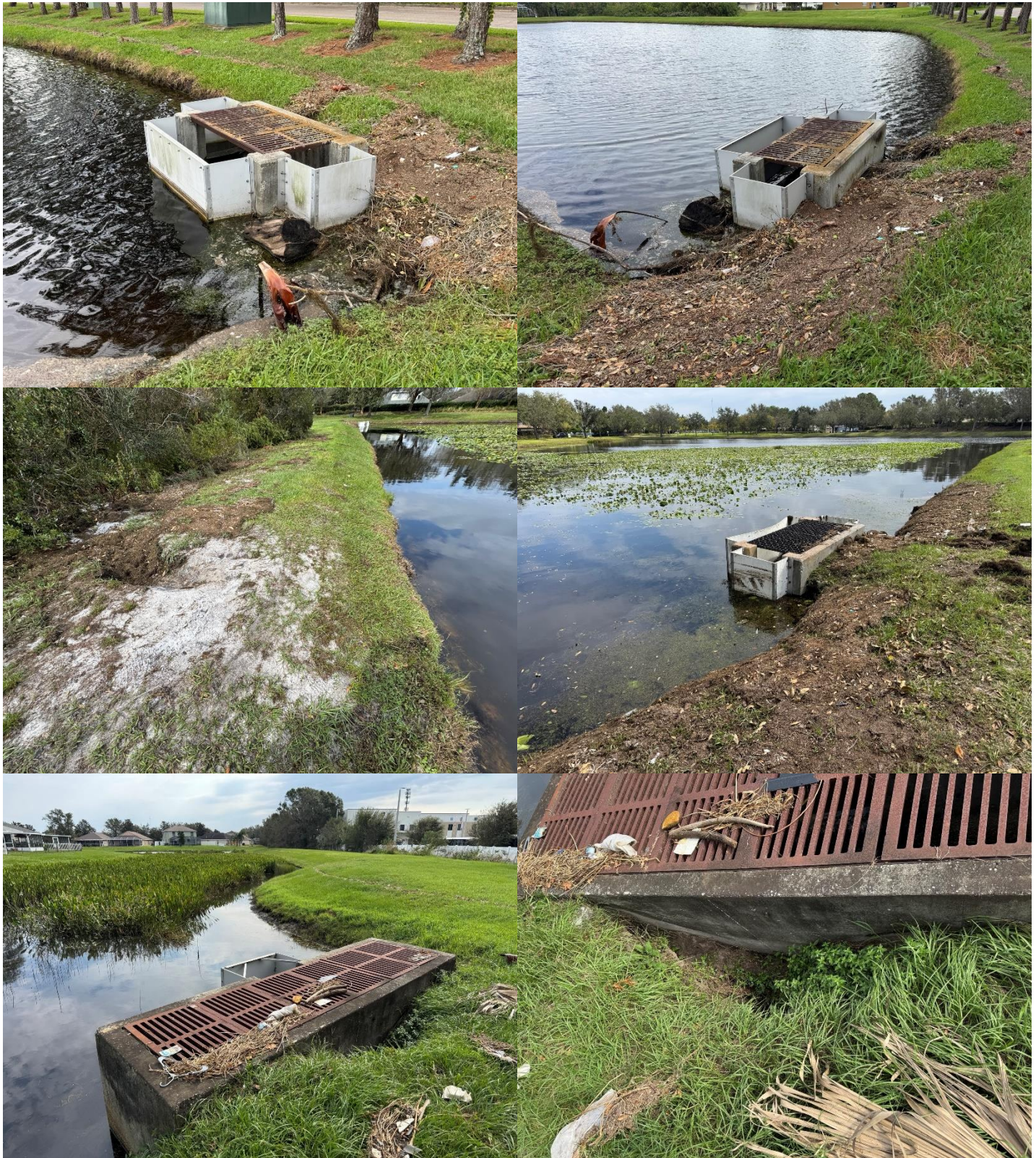
Photo 3 – Displays the erosion that has occurred at Pond 7, Pond 11, Pond FG and Pond 06 (severe case).
