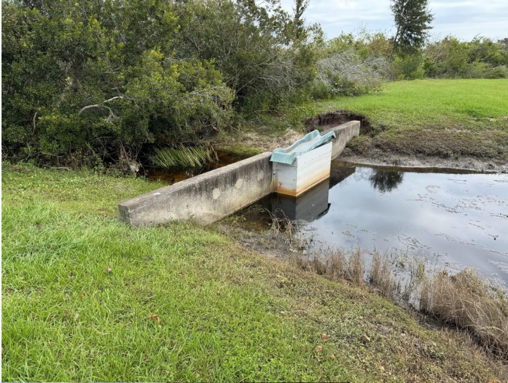
Photo 4 – Displays the failed weir structure at Pond LMA. The slide has been removed off the top of the structure.
